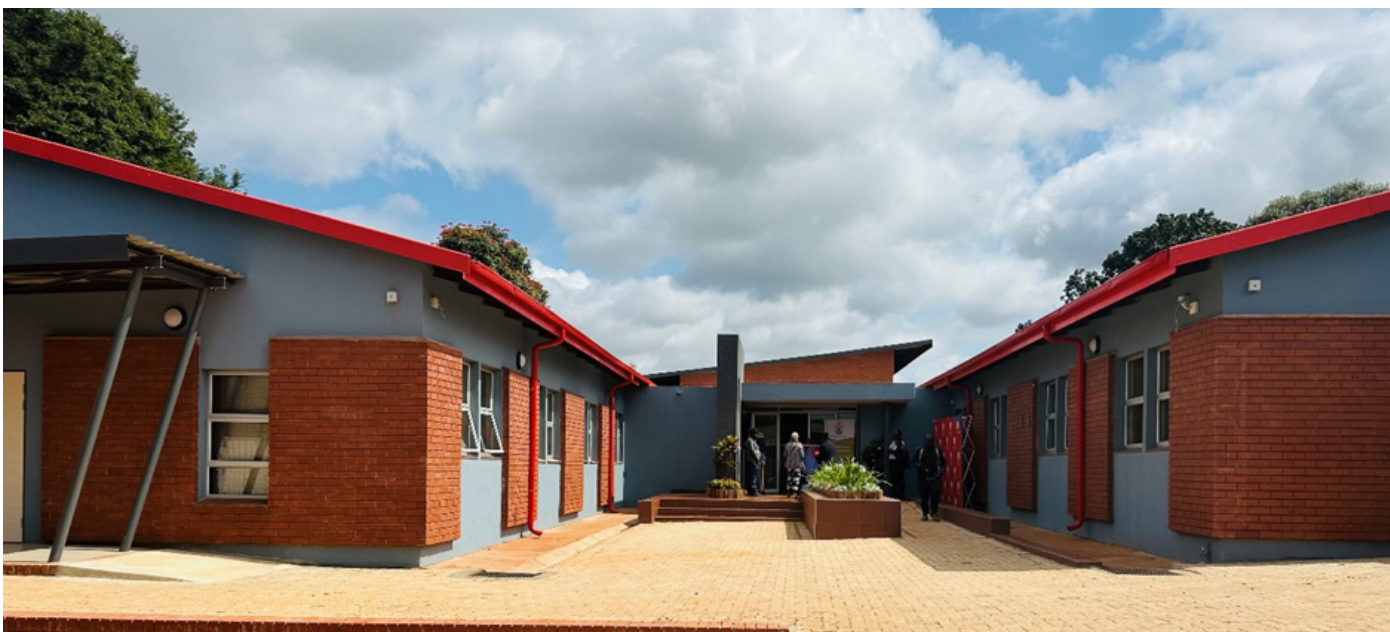
Recently completed DSU building
